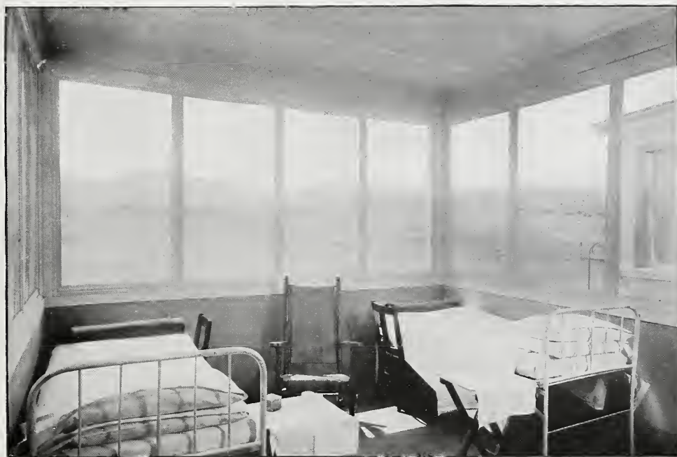
FIG. 181.—Sun porch, General Hospital No. 20, Whipple Barracks, Ariz.
